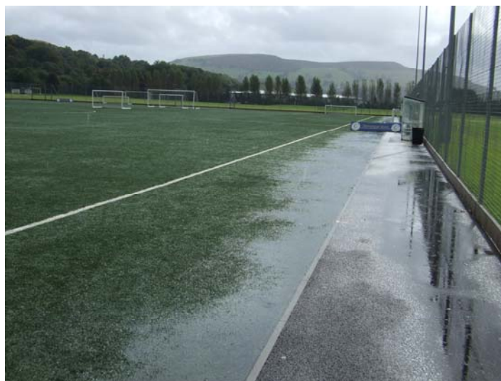
Figure 9. A waterlogged pitch at Tyn-y-Wern caused by heavy rainfall in December 2006.
