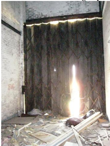
Plate 9: View of loading bay
