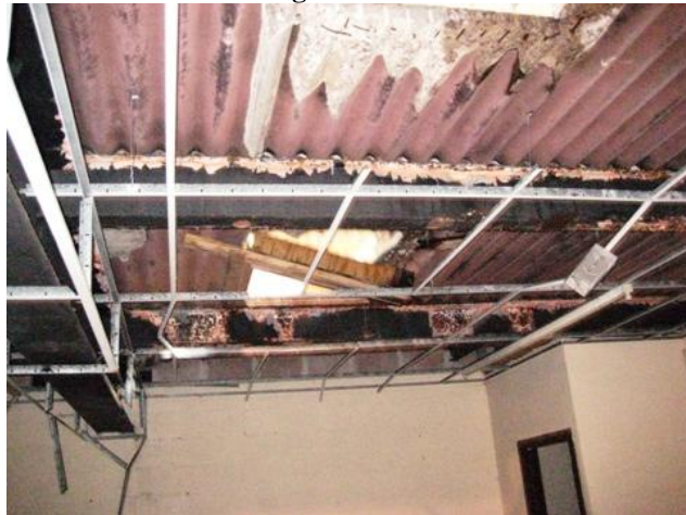
Plate 10: View of ceiling structure
